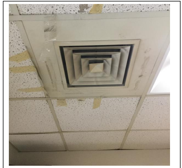
Taped supply vents
