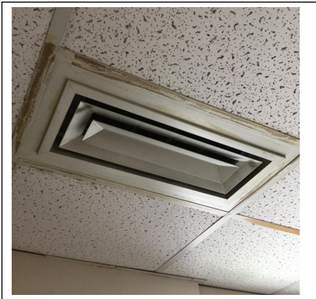
Taped supply vents
