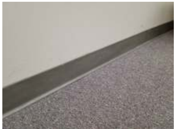
Photo #12 Non-asbestos containing 4" gray covebase and mastic (HA #8)
