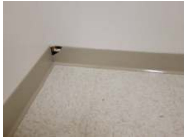
Photo #24 Non-asbestos containing 4" tan covebase and mastic (HA #18)
