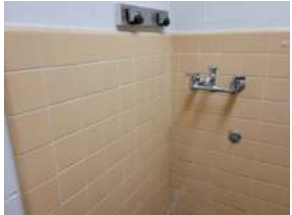
Photo #14 Non-asbestos containing ceramic wall tile grout and mortar (HA #10)
