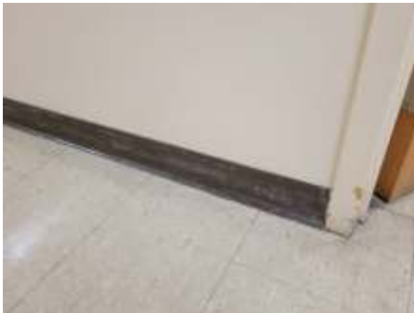
Photo #15 Non-asbestos containing 4" dark brown covebase and mastic (HA #11)
