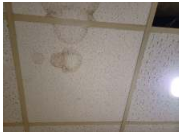
Photo #26 Non-asbestos containing 2' x 2' white ceiling tile with dots (HA #20)
