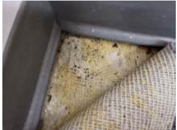
Photo #28 Non-asbestos containing tan carpet glue (HA #24)
