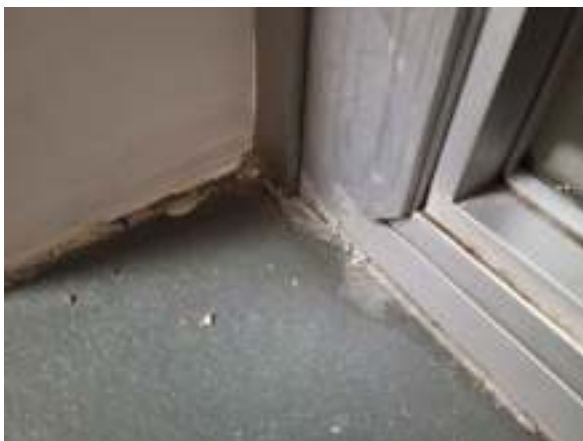
Photo #17 Non-asbestos containing gray interior window sealant (HA #13)
