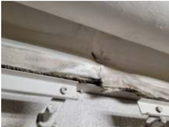
Photo #9 Non-asbestos containing white canvas wrap on HVAC duct (HA #5)
